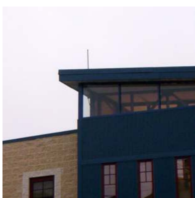
Figure 2 – Cisco Antenna Atop PEC's Family First Building
